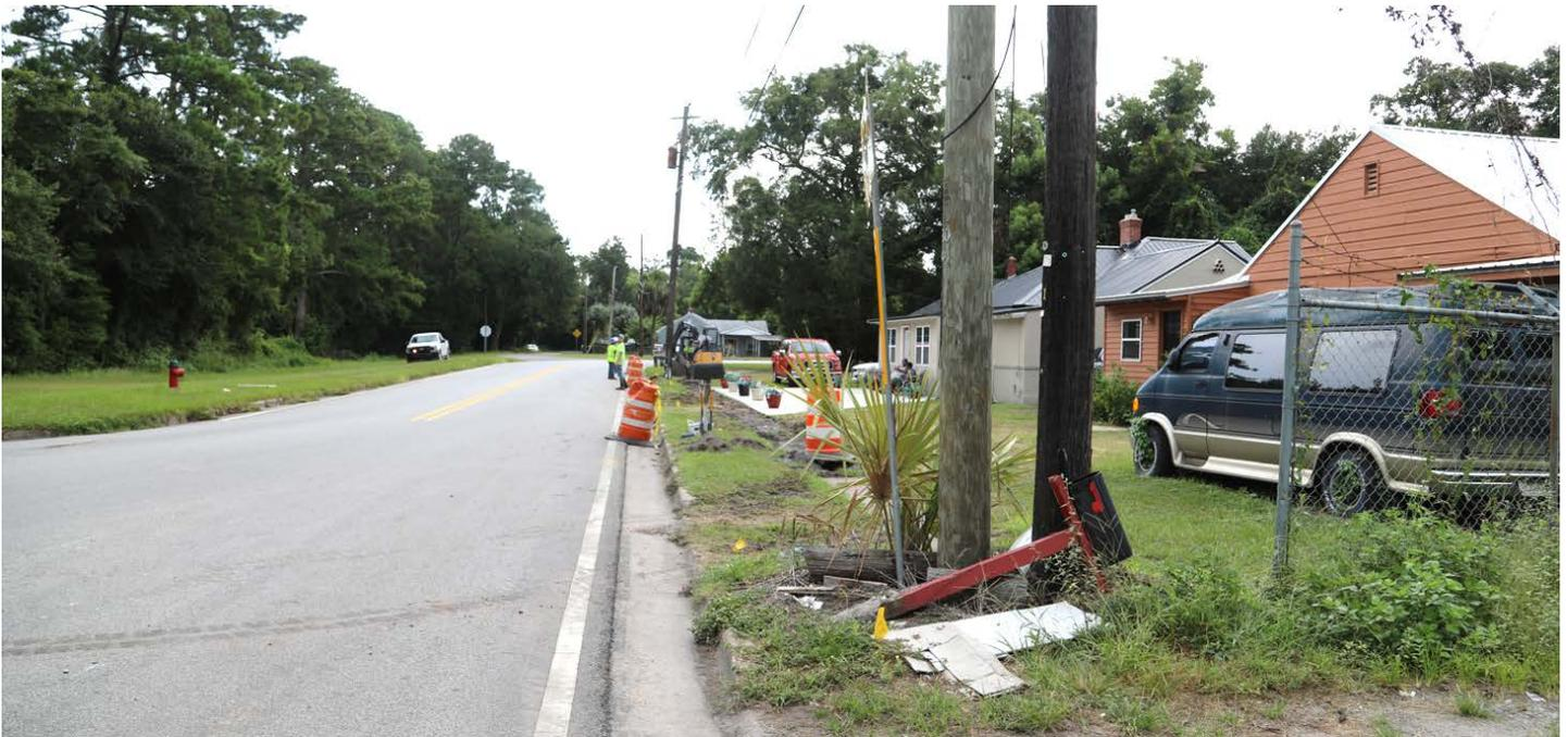
1. Sidewalk demolition and removal underway along Cochran Avenue in preparation for proposed watermain installation.
