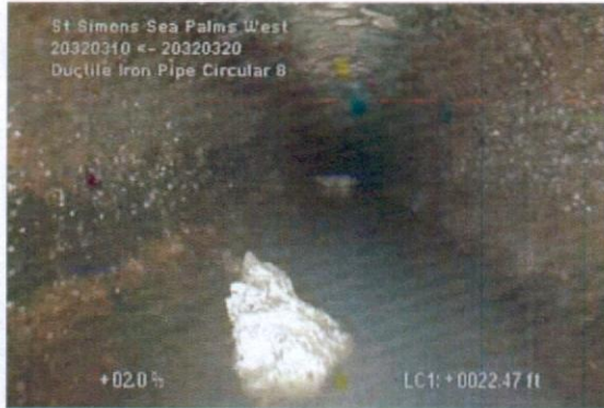
20320320+20320310_e1a50533-6f09-4024-b5b4-33bb82cfc6 b8.jpg, 00:02:36, 37.80ft Water Level, 35% of the vertical dimension
