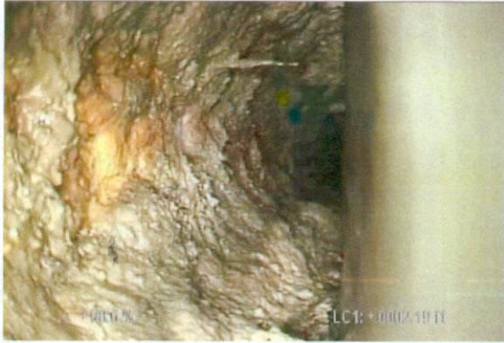
20320110+20320100_24f3b84a-7ff4-456c-ba16-8fb5cb33b64 f.JPG, 00:02:02, 2.10ft Survey Abandoned / Tuberculated Pipe
