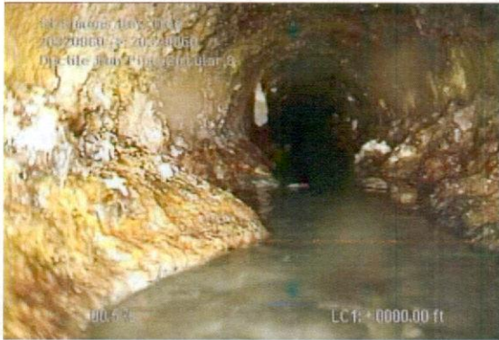
20320860+20320850_fa4fa195-62c2-4776-b60f-856e32cb14b c.JPG, 00:01:20, 0.01ft Survey Abandoned / Tuberculation
