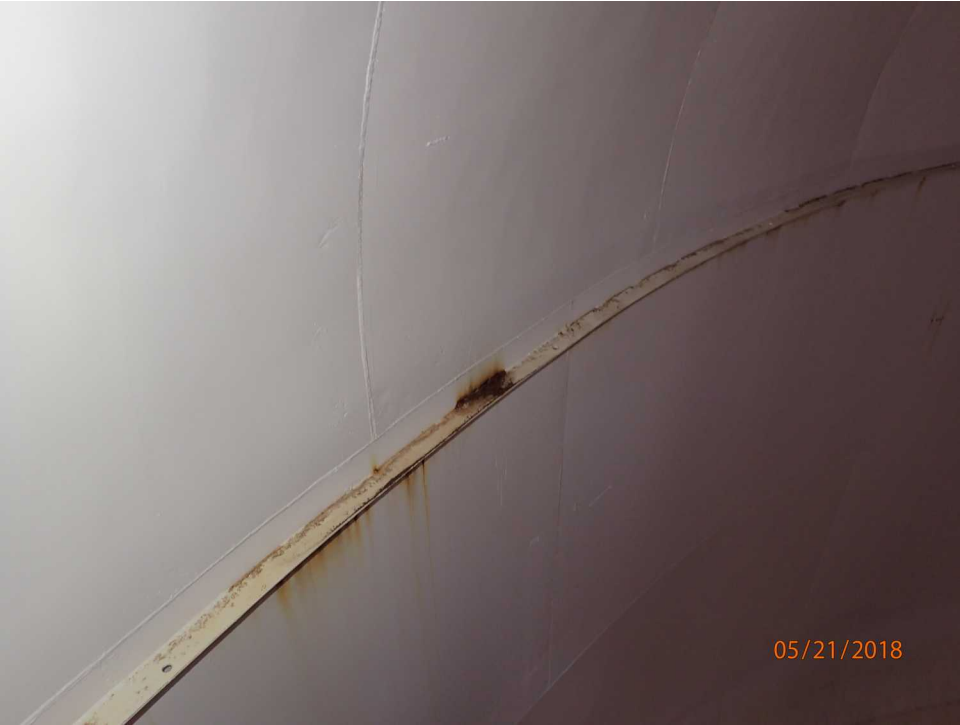
Rust on interior side angle
