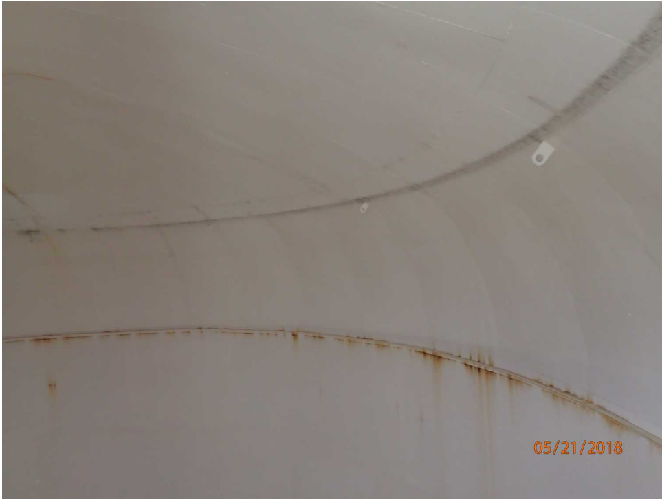
Rust on interior side angle
