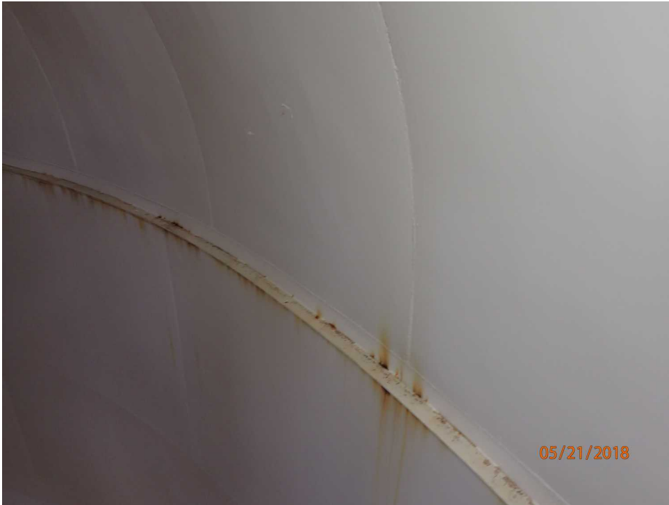
Rust on interior side angle
