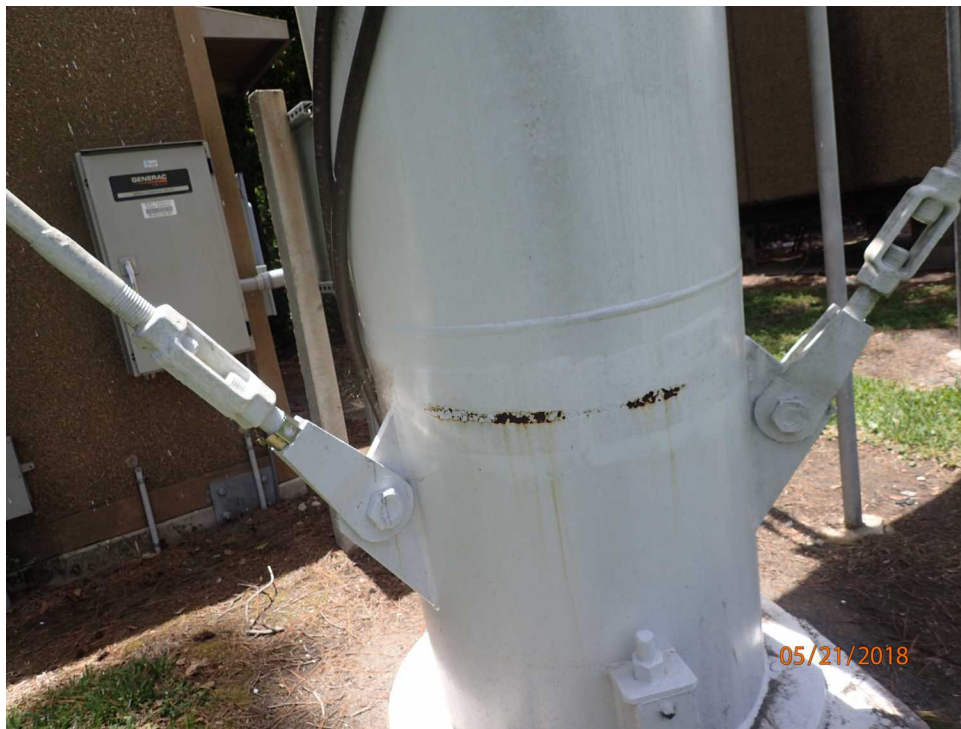
Rust spots on the bottom of the leg
