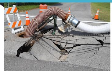
In April 2019, a large sinkhole developed on Whitlock Street due to a collapsed 30-inch concrete sewer pipe. The entire 540 feet of pipe that failed would require repair or replacement but the crews worked diligently to find a solution that would cause the least disruption in the area. Within a week, the entire pipe was repaired with a cured-in-place liner that hardens in the pipe to prevent further problems.
