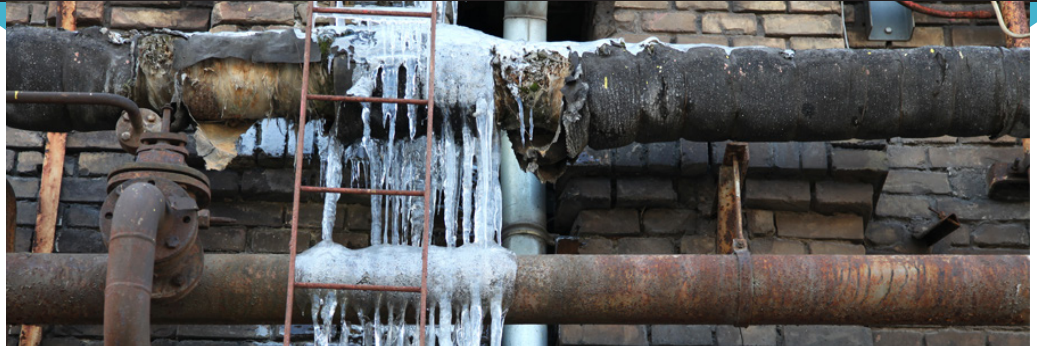
Insulate exposed pipes and fixtures to help ensure that your service isn't unavailable when freezing sets in.
