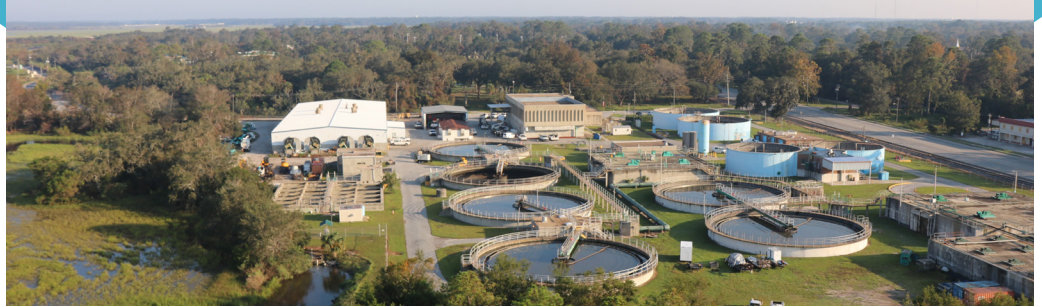
Aerial inspection by helicopter, courtesy of Sea Island resident Lance Toland, was performed on September 17, 2017 to determine any damages to the Academy Creek Wastewater Treatment Plant caused by Hurricane Irma.
