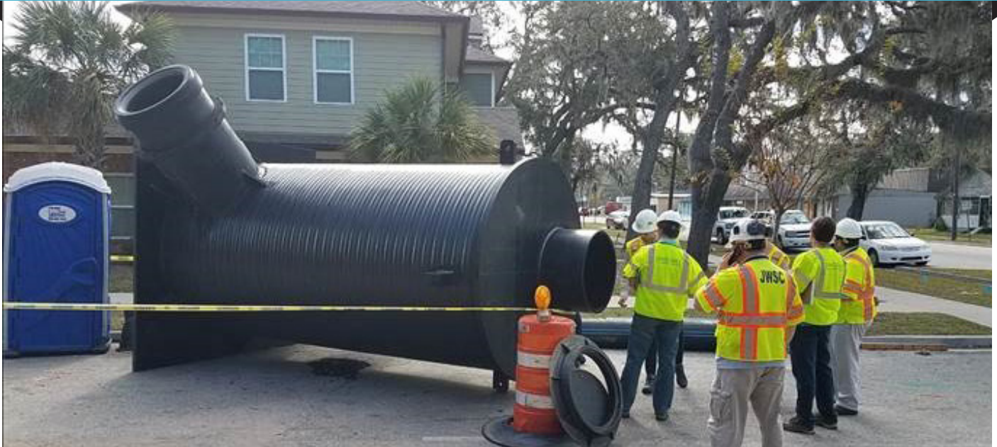
In mid-December, BGJWSC staff monitored the installation of a new manhole in front of Norwich Commons at Norwich and 5th St. This High Density Polyethylene (HDPE) plastic manhole is the first of its kind in Glynn County.
