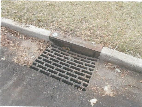
Drainage Along Atlanta Avenue At Frontage
