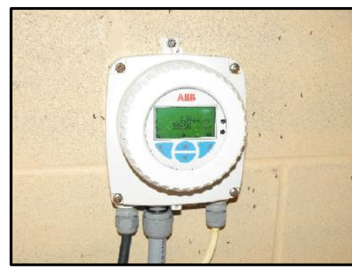
FLOW TRANSMITTER FIT-1 TO BE RELOCATED N.T.S.
