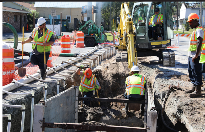
Sewer Main Repairs at MLK and G Street - 10/26/17
