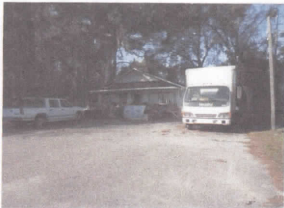
Commercial Building Adjacent To East Of Subject
