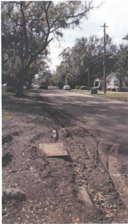
I St & Wilson Ave. Intersection (01.04.17)
