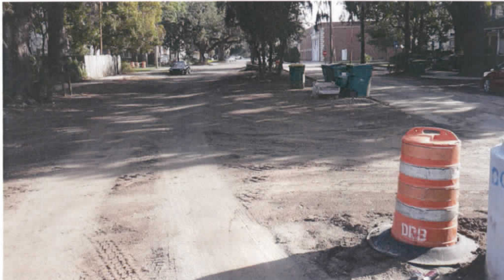
Re-addressing the roads on Mansfield St. (01.04.17)
