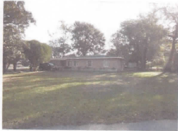
Single-Family Home Adjacent To West Of Subject
