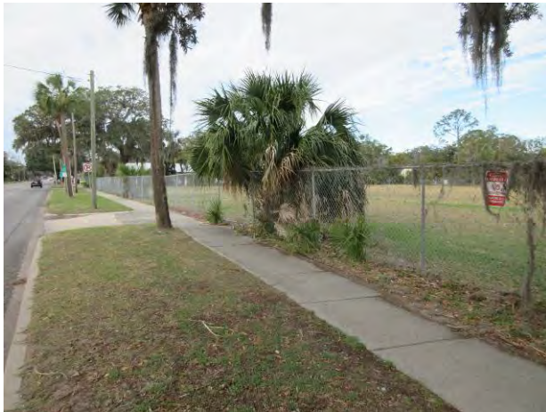
Sidewalk And Fence Along Gloucester Street Frontage
