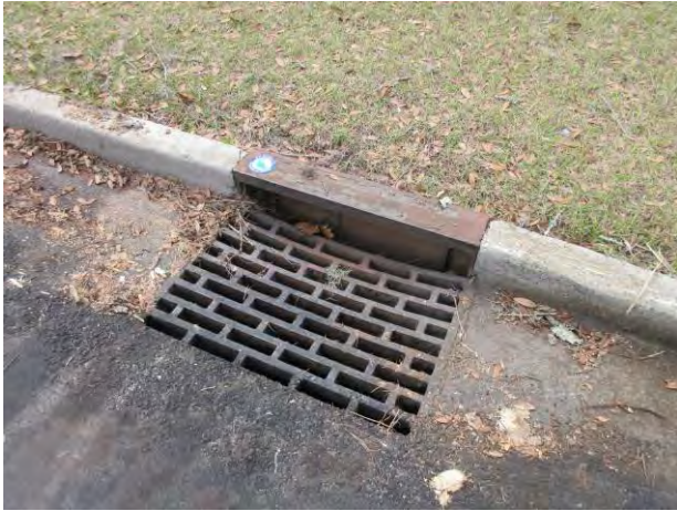
Drainage Along Atlanta Avenue At Frontage
