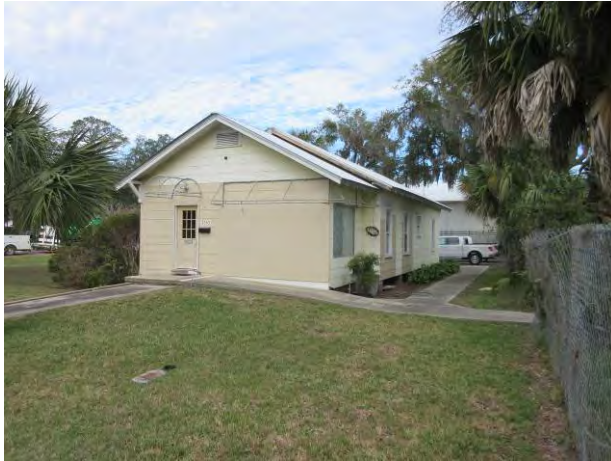
Former Residence, Current Office, Adjacent To West Of Subject
