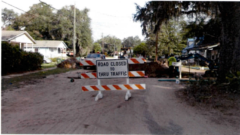
Installation of sewer services
