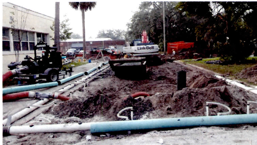
Installation of Manhole along Richmond St.
