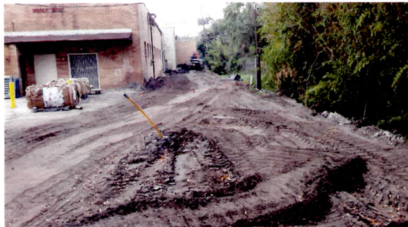
Sewer Main installation behind Lanier Plaza
