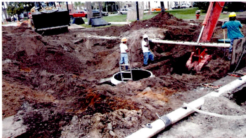
Manhole Installation at intersection of Richmond St and Mansfield St.
