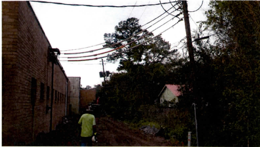
Existing overhead utility conflict
