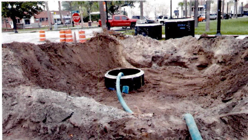
Manhole installation at intersection of Mansfield St. and Newcastle St.
