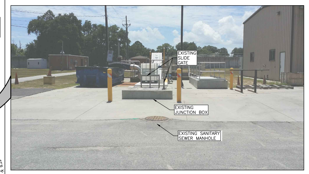
LOOKING SOUTH TOWARDS EXISTING JUNCTION BOX BYPASS POINT
