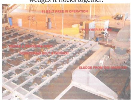
There is just enough Polymer added to make the sludge flock after the fourth row of wedges.
