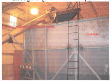
The Hopper is our storage area for the sludge cake. The dryer holds six tons per load and the hopper is a 50 yard container, this is enough for 5 loads.
